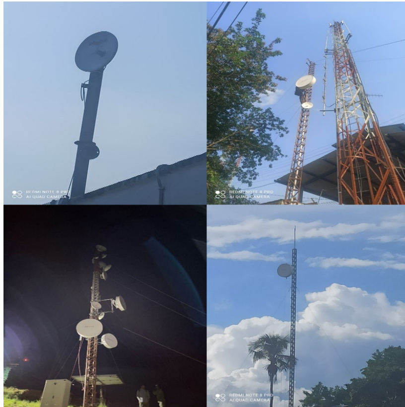
Figure 2. Installation of the system antennas.
